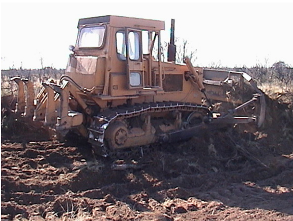
Fig. 2. Crawler tractor used for land clearing.
