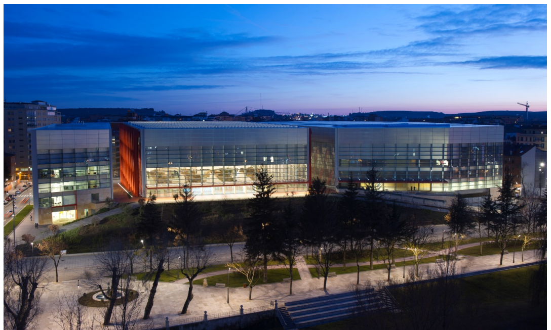
Figure 2. External view of the MEH building. Source: MEH.
