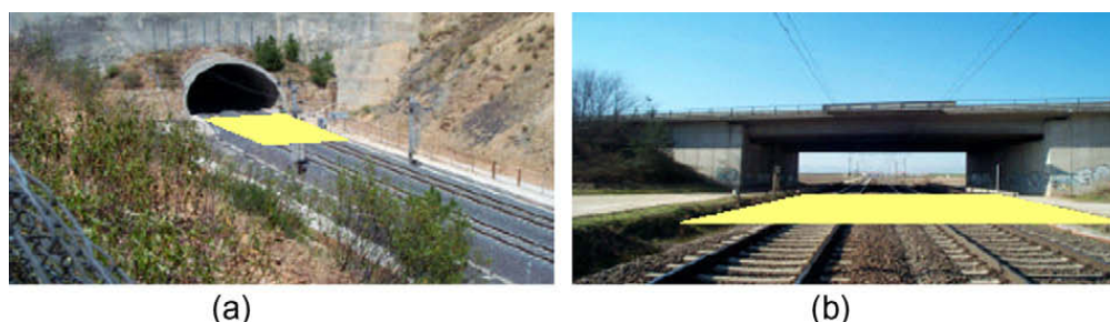
Fig. 2. Critical zones: (a) tunnel and (b) overpass.
