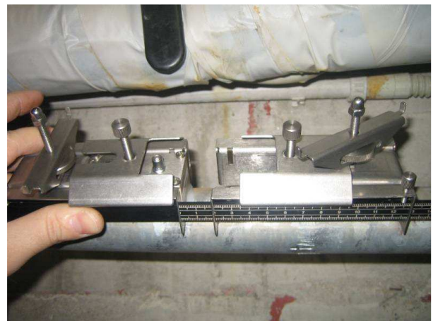
Fig. 2. Installation of flow meter
