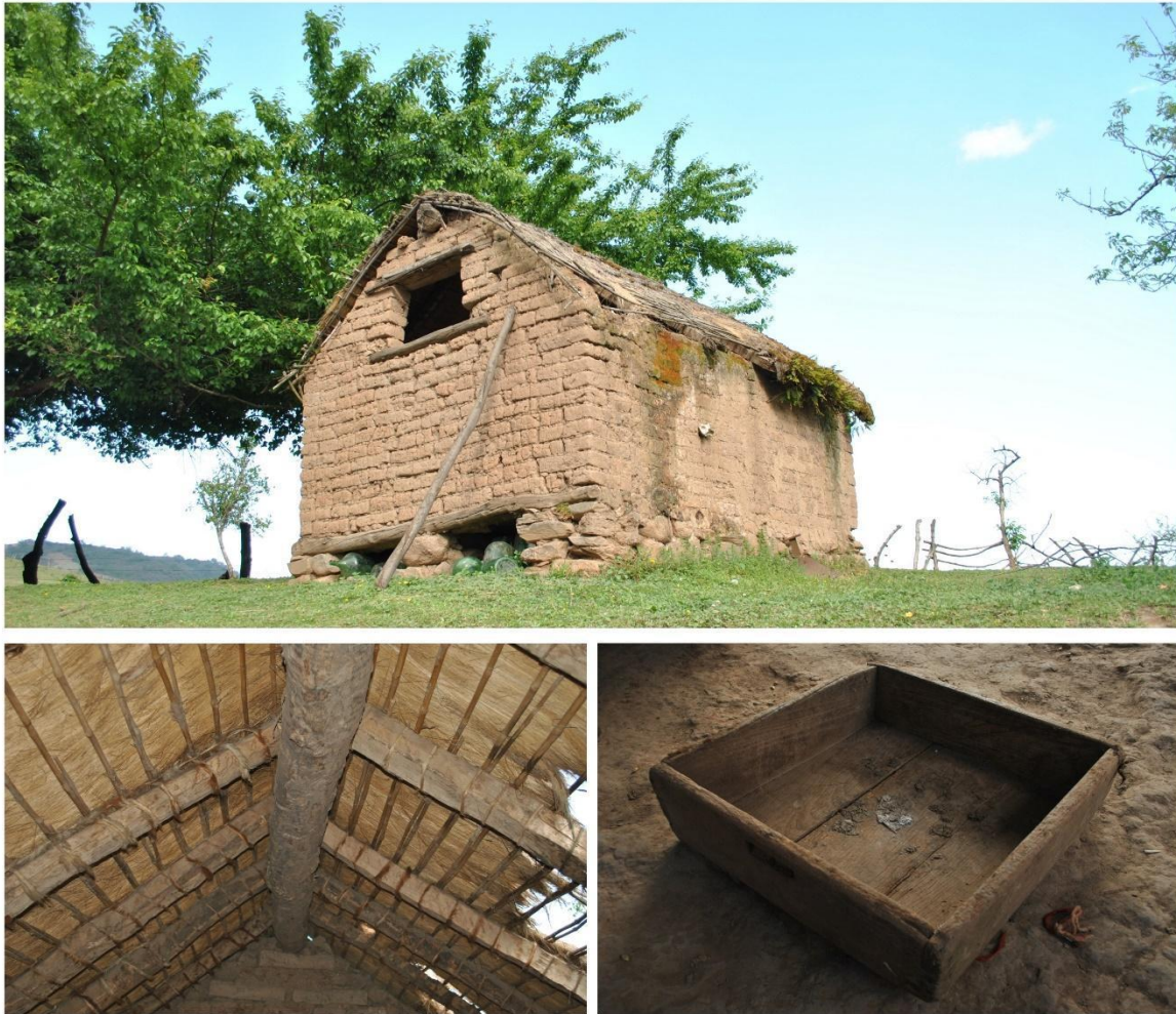
Figure 7. “Pirhua” storage structure in Flora’s house, constructed with perishable material (adobe, aliso timbers, cane, and thatch). On the right bottom, a talmud to calculate the amount of Zea mays to exchange (Photographs by J. Salazar).
