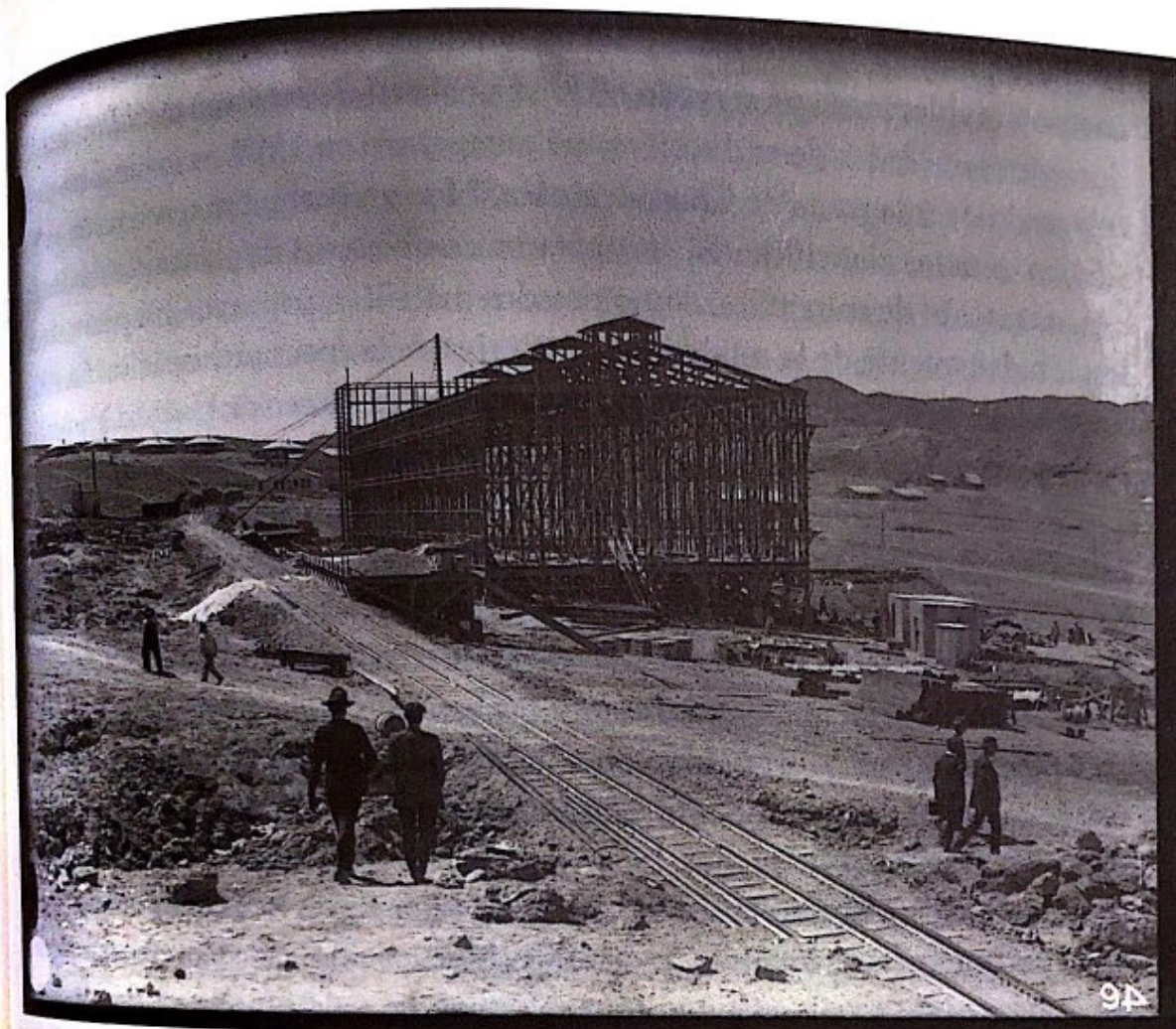
Figura 3. Estanque de preparación de ácido. Chuquicamata. C. Glover, "Glass slide #94" [Placa de vidrio #94], ca. 1913-1914, en Railroad construction and mining in Bolivia and Chile , Getty Research Institute, Los Angeles (90.R.51).
