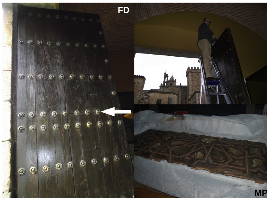
Fig. 4. The front door (FD) from the Las Veletas palace (Cáceres, Spain) constructed with the original wood pieces dated to the period 1562–1717. The arrow indicates the latest restoration of the lower part in 1872, showing the replacement of the wood material. The medieval city of Cáceres can be seen in the upper right part of the image. A Mudejar panelling (MP) covering the period 1658–1698 ( r = 0.71 ) is shown.
