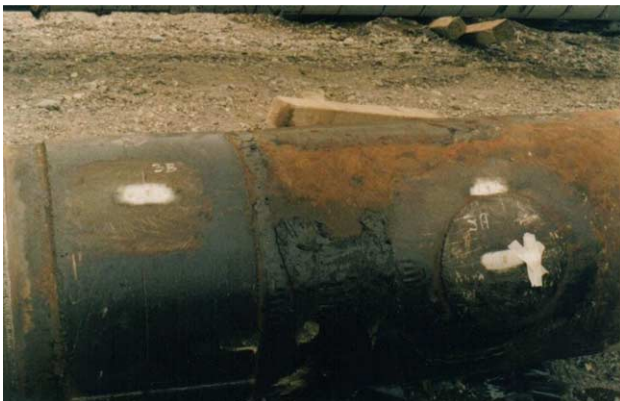
Fig. 3. Repairs installed in pipe 1: a circular patch and a sleeve reinforcement.
