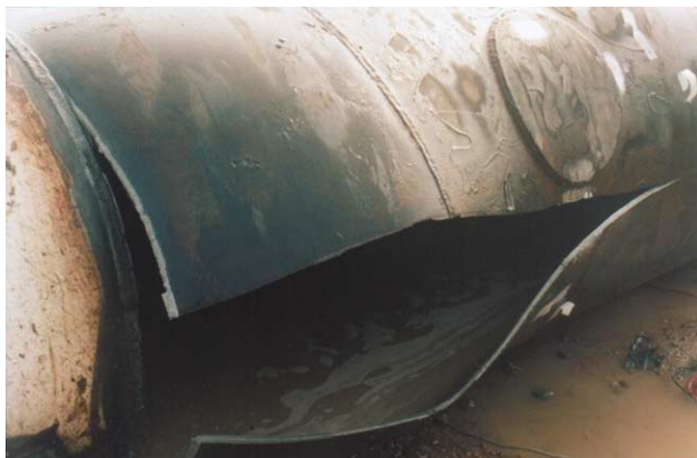
Fig. 6. Circular patch in pipe 4 (repair 4A).
