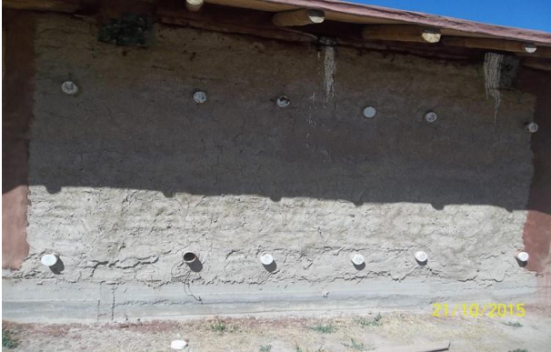
Figure 12: The Trombe-Michel wall without its external glazing and with PVC pipes as air vents.
