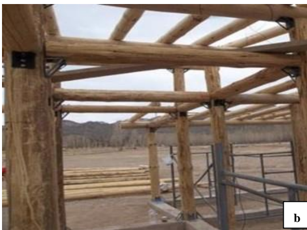
Figure 9: a- St. Andrew's cross on walls with cane struts b- Main structure with columns and wooden beams.
