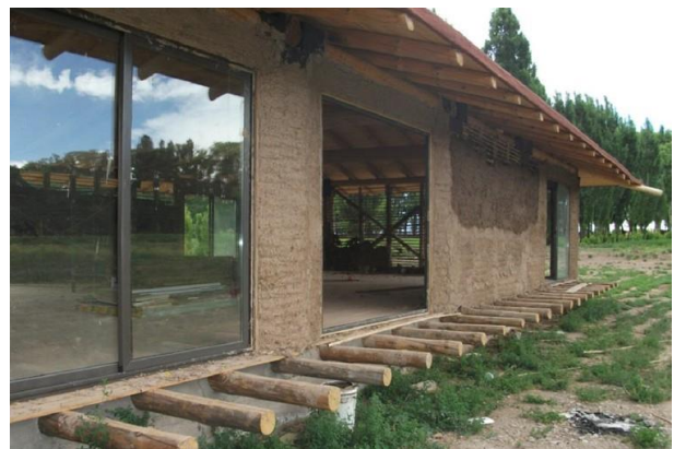
Figure 11: 60cm-wide eaves protect the "Quincha" walls from the rain
