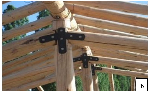
Figure 10: a- Metal plate connecting timber joints at floor level. b- Metal plate connecting timber joints at ceiling level.
