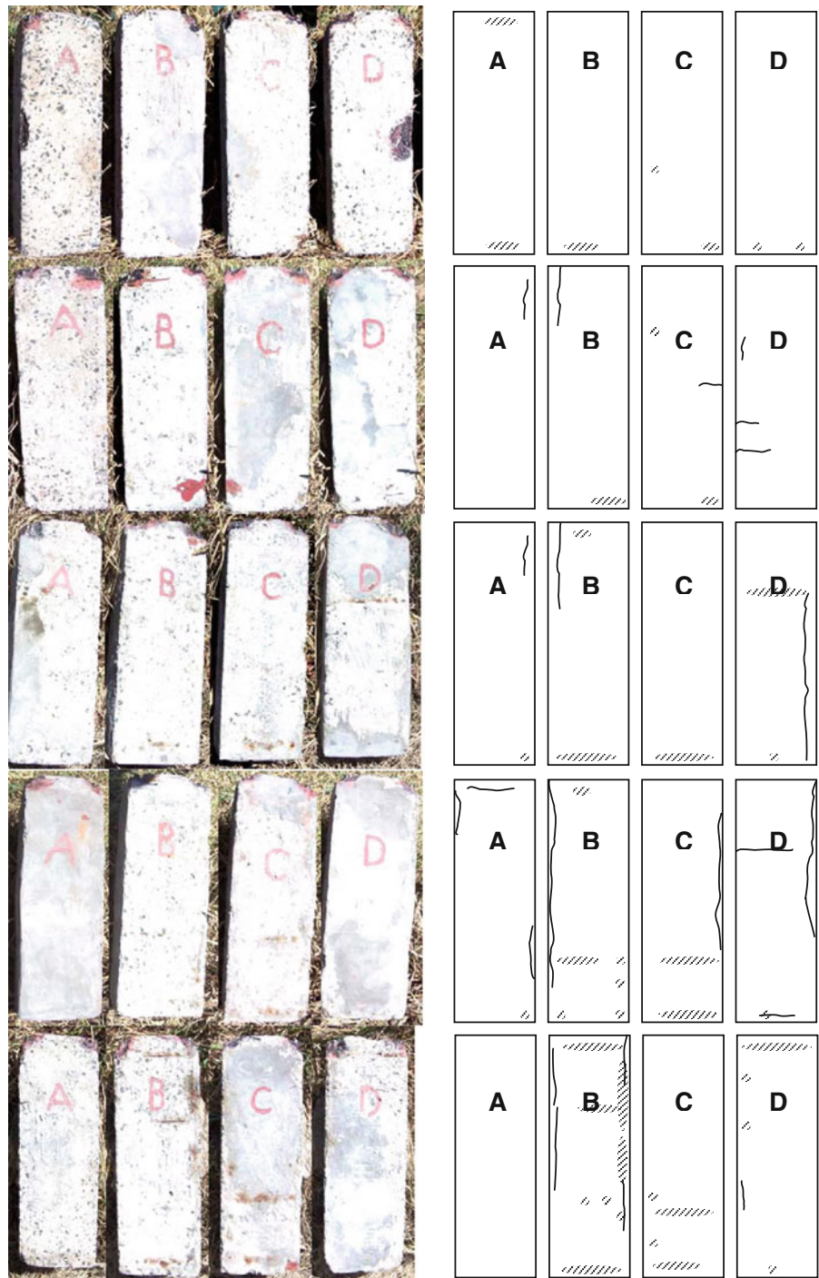
Fig. 10 Cracking patterns and rusting on reinforced concrete members
