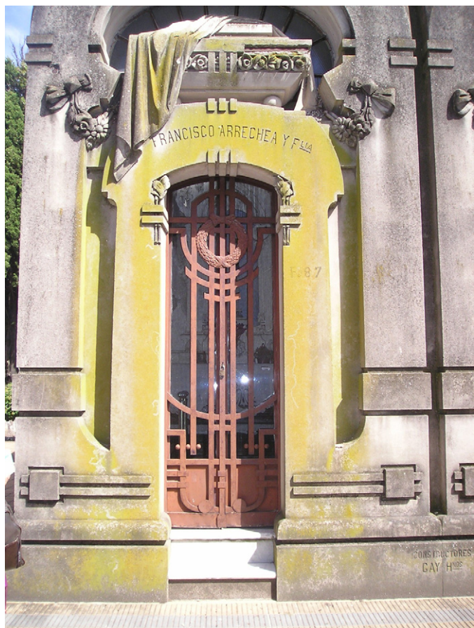
Fig. 1. Portico of the crypt of Francisco Arrechea (crypt F87), which is of architectural interest because of its Art Nouveau style. The yellowish coloration is indicative of the presence of Caloplaca austrocintrina .
