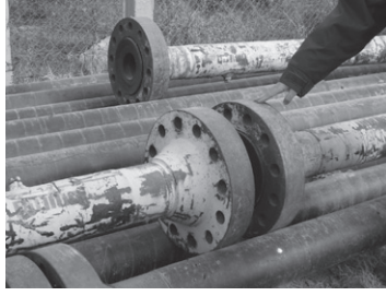
Figure 1. A pipe flange similar to those we looked for.
