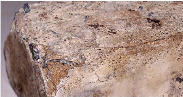
Fig. 4. Longitudinal cracking near the edges of adjacent faces.
