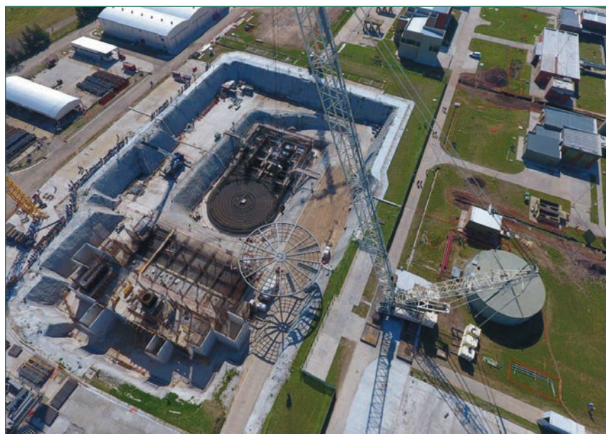
Figure 6. Details of the ongoing construction: first stage of the liner placement.
