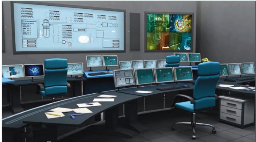
Figure 4. Control room with a distributed software system.
