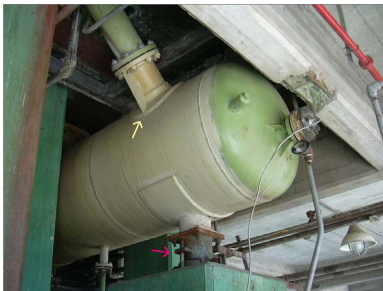
Fig. 1. Case 1: Elastics supports of discharge vessels.
