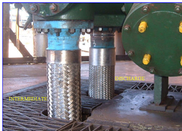
Fig. 2. Replaced flexible at discharge and intermediate pressure.
