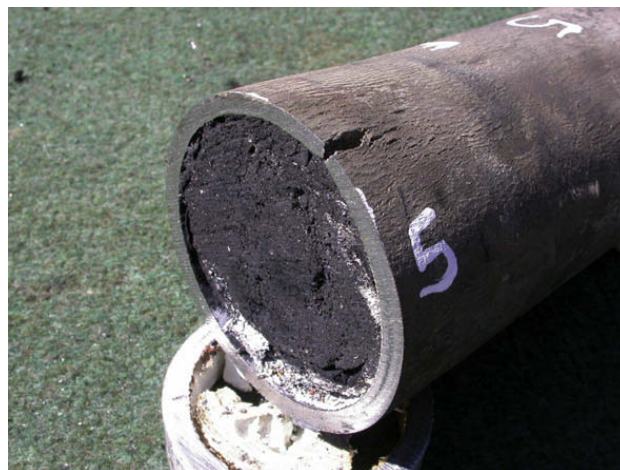
Fig. 3. Carbonized polymer clog in the failed section.
