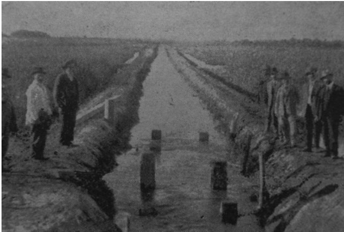
Figure 4. The Tulumaya Canal, Built by Land Owners, Mainly European Immigrants, to Drain the Tulumaya Wetlands
