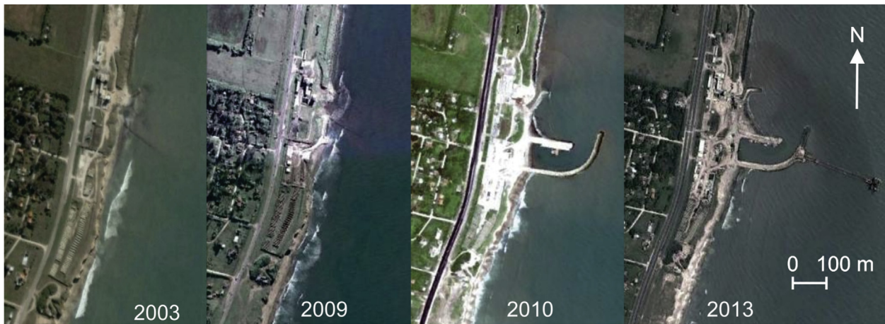
Fig. 7. To fix the stability of the outfall pipeline in Camet, two jetties were constructed.
