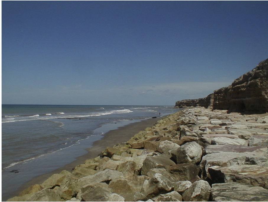
Fig. 10. Rock revetments protection the foot of sea cliffs at Mar del Plata. Sand accumulates at the foot of the ripraps during the summer season.
