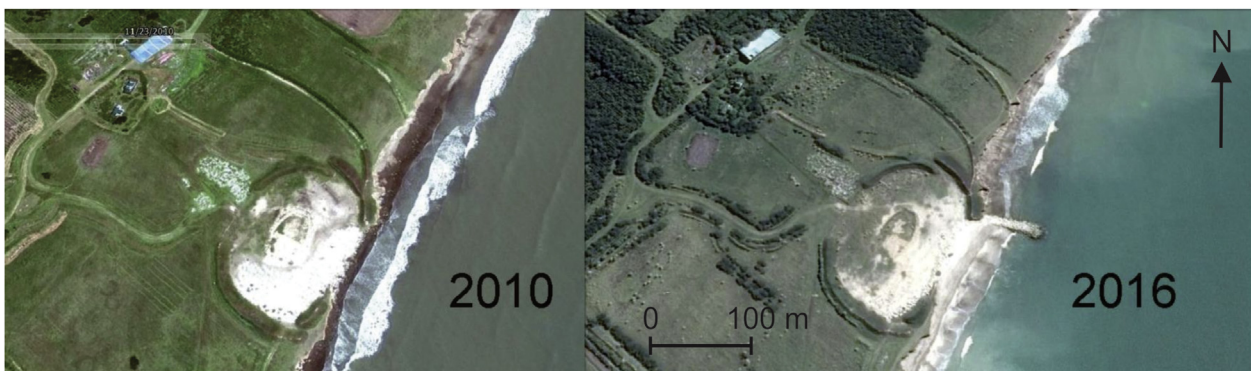
Fig. 9. Clandestine groin constructed at San Manuel Estancia.
