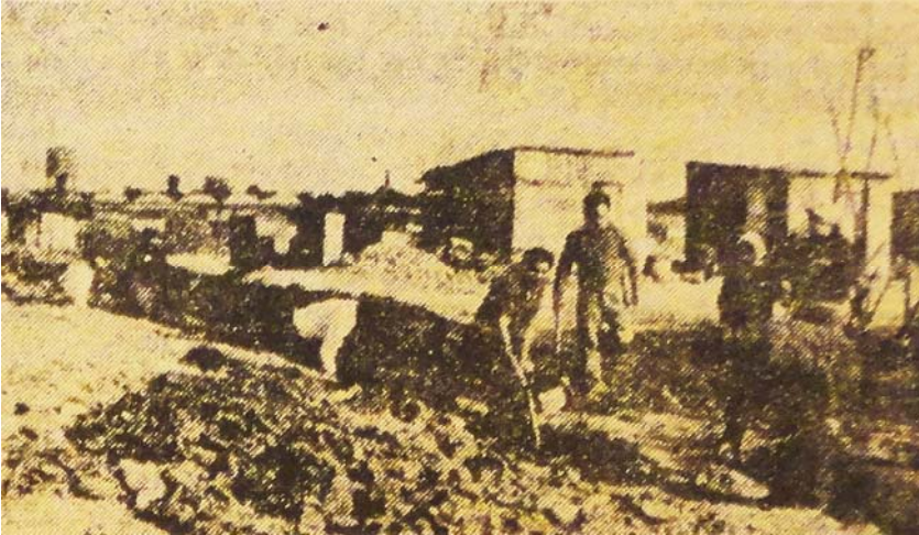
Figure 1. Residents of Villa Rotonda Varela opening trenches for fresh water pipework. Source: La voz de las villas , February 1965.
