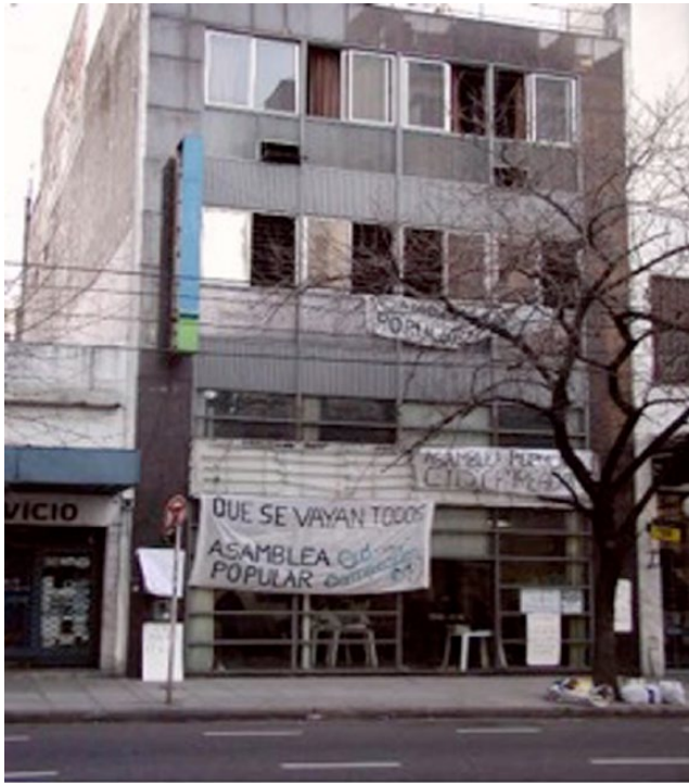
Figure 2. Cid Campeador House, headquarters of the Cid Campeador Popular Assembly in 2002 (courtesy of a member of the assembly).
