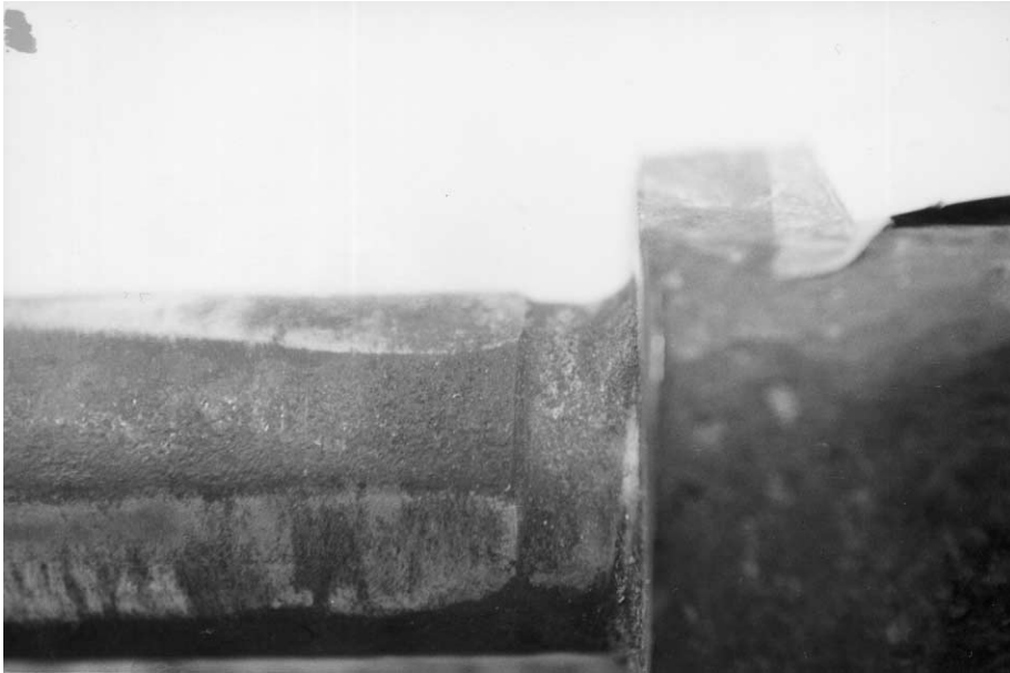
Fig. 10. Evidence of high premature wear in the eye to bolt weld, due to friction against the walls of its lodging in the A-frame.
