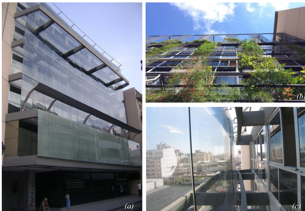
Fig. 4. Building facades. (a) West DGF façades, one-storey ventilated DGF at the first floor and multi-storey DGF (2nd to 5th floor). (b) East green wall façade. (c) air cavity of the multi-storey DGF where the screen printing in the outer glass is visible.
