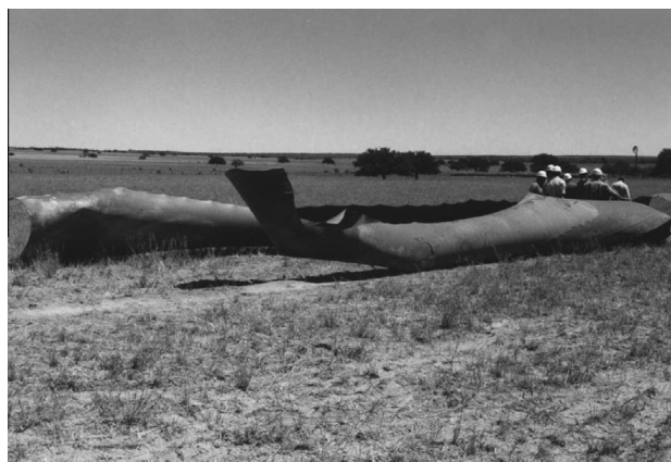
Fig. 2b. Failure in a natural gas pipeline [4].
