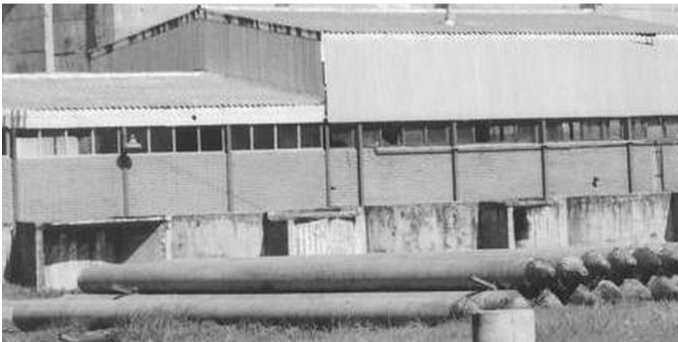
Figure 3 Concrete annular piles tested in CTNOA S.A.
