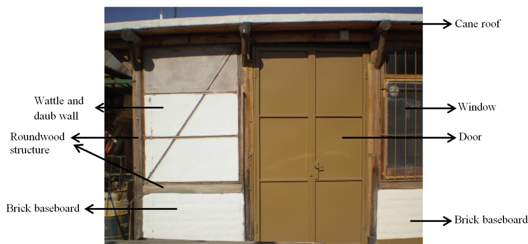
Figure 1. Wattle and daub constructions parts
