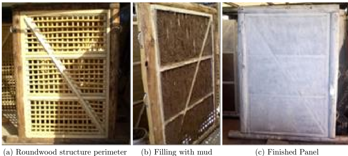
Figure 4. Assembly's sequence of wattle and daub
