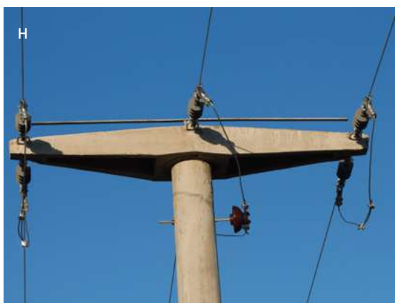
Figure 189. E: An electrocuted variable hawk in central Argentina on a pole combining wire jumpers above the crossarm with a dangerous construction material (steel-reinforced concrete). F: Black-chested buzzard eagle flying from a retrofitted pole where jumper wires were moved below the crossarm to reduce electrocution risk. G and H: Bird-friendly pole designs over 40 km of a newly built power line in Argentina. © José Hernán Sarasola and Maximiliano Galmes/CECARA
