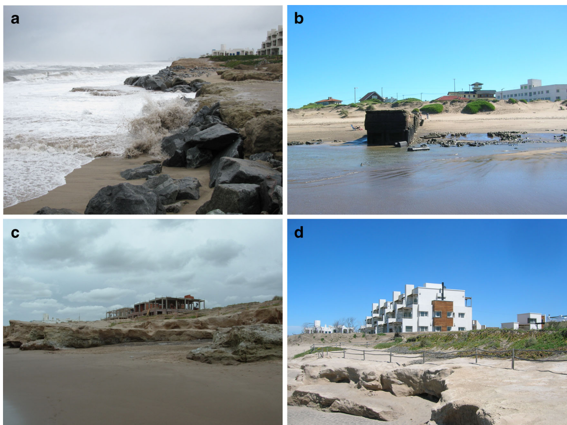
Fig. 5 Areas with high coastal erosion risk. a Waves reach the urbanized cliff toe during storms in Bahía de los Vientos (22-07-12) b A rigid structure in front of a sector in Costa Bonita at low tide (18-03-08) c
