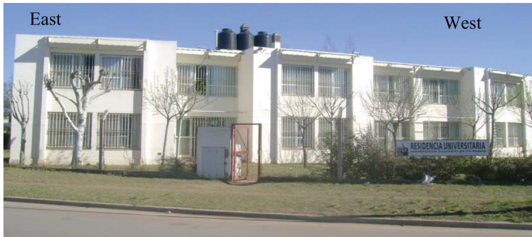
Figure 3 • Building's facade facing north and the location of the apartments.
