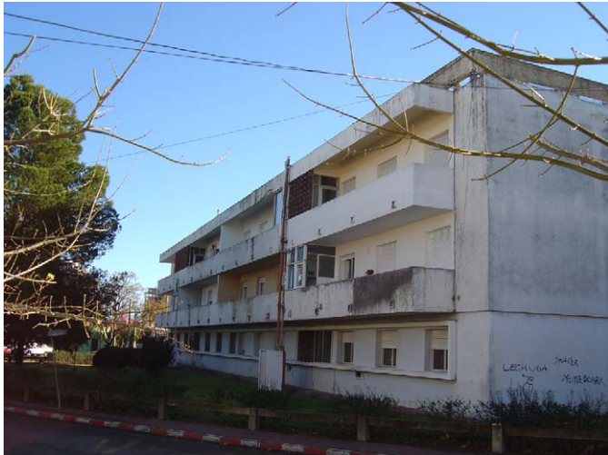
Fig. 8. Building's south facade (block 74).
