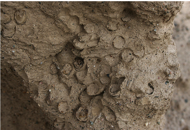
Fig. 3. Arrangement of cells and cavities in the wall.
