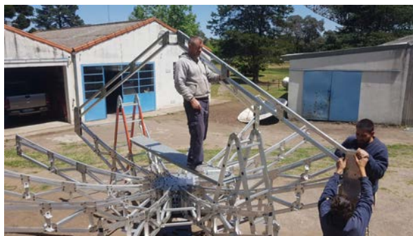
Fig. 12. First parabolic dish under construction.
