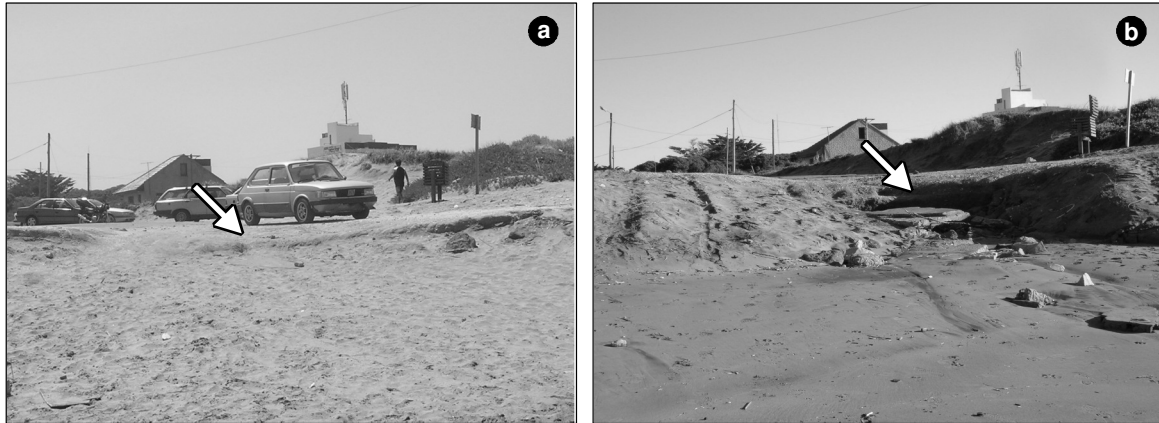
Figure 5. San Martín Ave. viewed from the beach: (a) January 2007 and (b) April 2007. Observe the rubble and the decrease in beach level.
