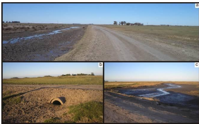
Figure 4. (a) Photo of the marsh area in which an internal road lacking drainage blocks the tidal flow towards the marsh section to the right of the image; (b) internal road with blocked drainage pipes; (c) tidal channel intersected by an internal road with no drainage.
