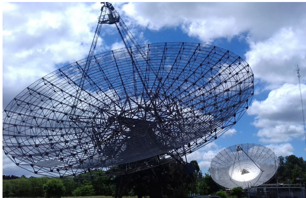
Fig. 1. View of IAR antennas, A2 (left) and A1 (right).
