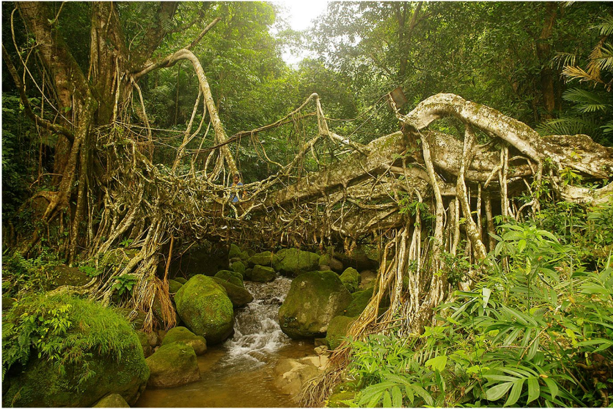
Fig. 1 Living root bridge in Cherrapunji in North-East India. (Photo by Arindam Das, CC BY-SA 4.0 < https://creativecommons.org/licenses/by-sa/4.0/ >, via Wikimedia Commons)
