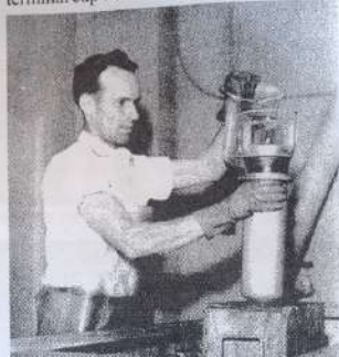
Fig. 8. Washing the anode assembly
