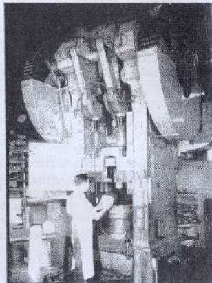
Fig. 1. Forming the anode
