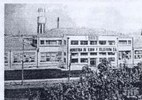
Fig. 2. IRT plant in Santiago, 1975
