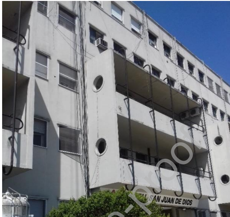
Fig. 10. North façade of Instituto del Tórax pavilion
