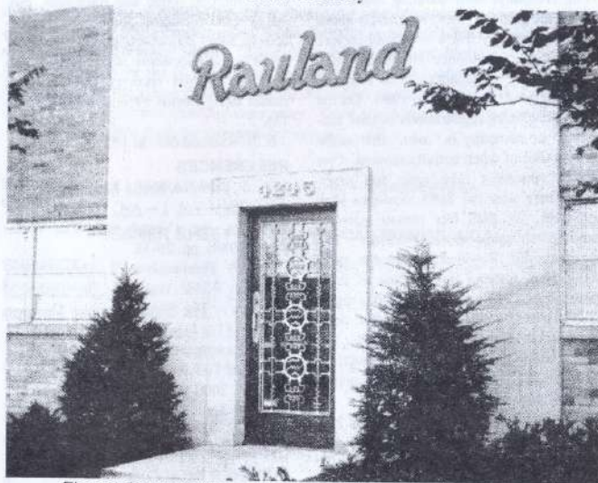
Elegant doorway at the entrance to the Knox Ave. plant, ca. 1943.
