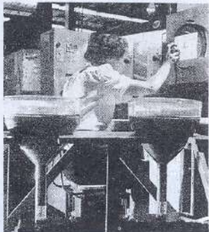
Making final tests on 10-inch kinescopes using a special chart as a reference standard.
