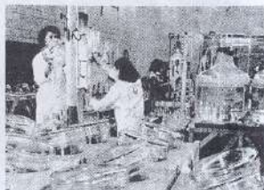
Operators prepare the fluorescent solution which forms the picture screen.
