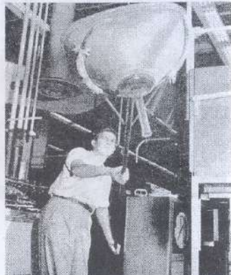
This fork-like instrument, guided by a worker, lifts a hot tube onto a cooling belt.
