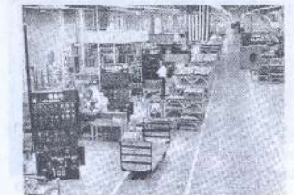
Racks of cathode-ray tubes move down one of the production lines.
