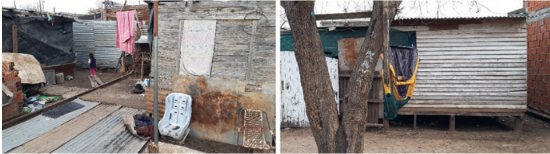
Figure 9: Precarious construction of houses and construction on stilts after the 2012 flood (Photos by the author)
