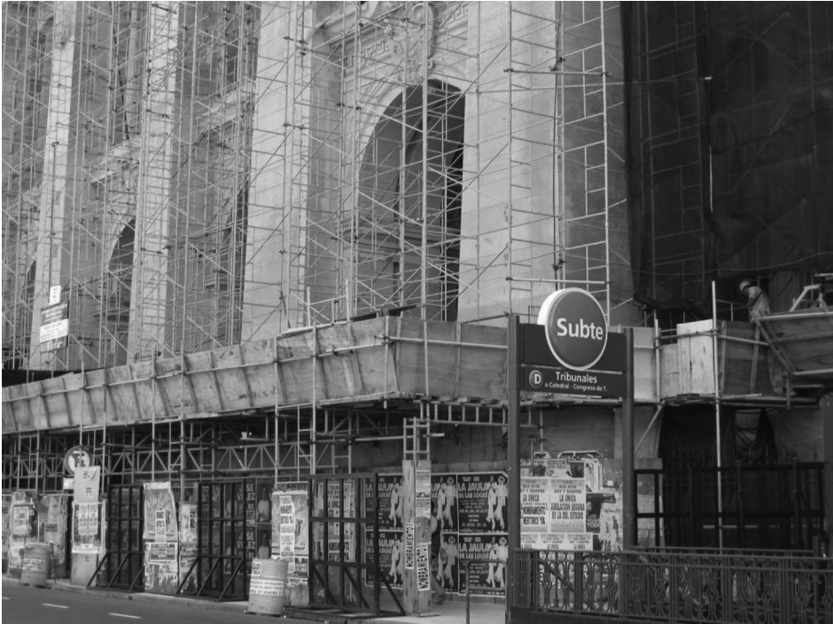
Figure 1. Restoration works on the Palacio's front façade, Buenos Aires, January 31, 2007
