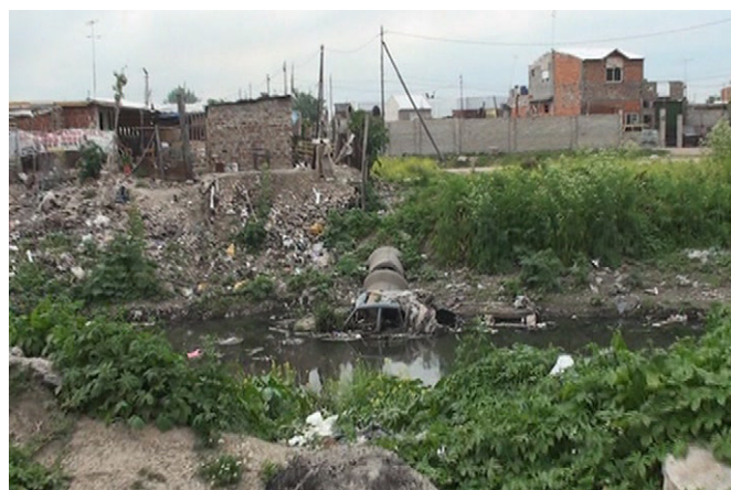
Fig. 4. The creek at the heart of the shantytown, rendered what the neighbors call zanjón . Note the pipe drainage outlet.
