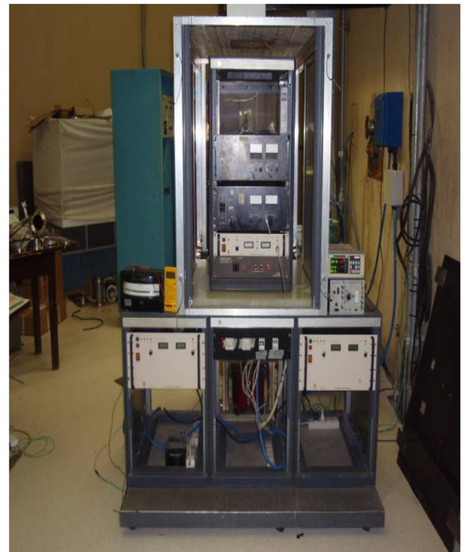
Fig. 4. Front view of the test stand, displaying the two 50 kV, 60 mA high voltage supplies (bottom panels) used for polarizing the ion source and an extraction electrode. Within the upper grounded Faraday cage one sees other power supplies for filament and gas discharge mounted on an insulated platform.
