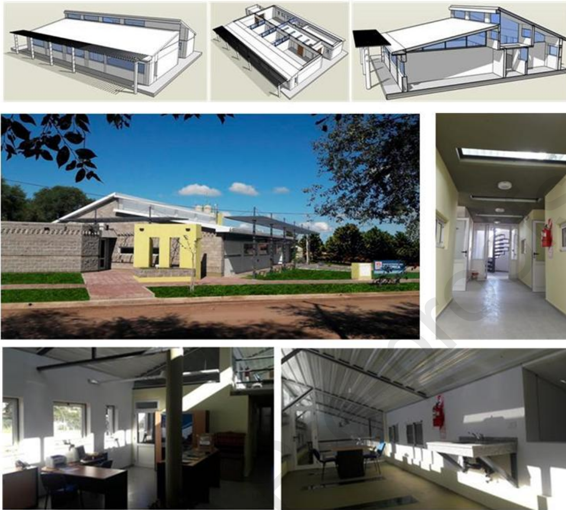
Figure 5: Plant and volumetric configuration. References: 1- Entrance, 2- Administration, 3- Technical office, 4-Meeting room, 5- Director's office, 6- Circulation, 7- Service, 8- Multipurpose room, 9- Access to technical-thermal plenum, 10- technical-thermal plenum. North-facing and passive solar heating; Administration, Technical plenum, and corridor between areas with and without direct solar gains. The photos were taken on July 15 between 14hs and 15hs.
