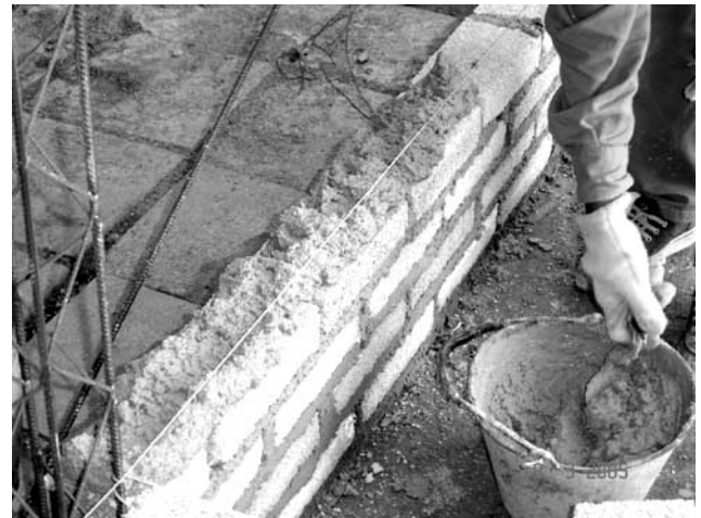
Fig. (6). Wall masonry constructed with bricks made of recycled plastics.
