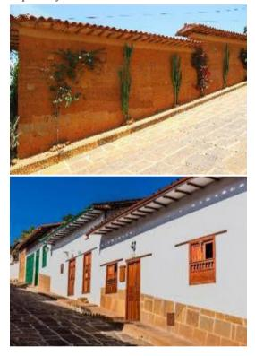
**Figure 2.** City of Barichara in Colombia. Constructions with rammed earth walls <sup>[6]</sup>.
