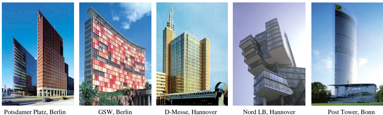
Figure 1. Some typical examples of the 30 buildings chosen for this field study.
