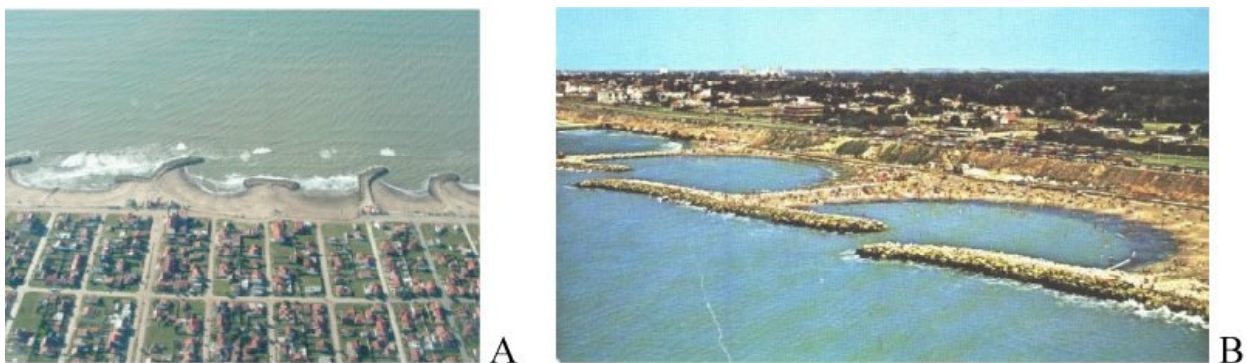
Figure 2. Hard structures north of Mar del Plata (Camet). A. Groins (straight and bended) cause longshore-drift obstruction; B. T-groins cause wave diffraction, induce sand sedimentation but impede the renewal of water at the compartments.
